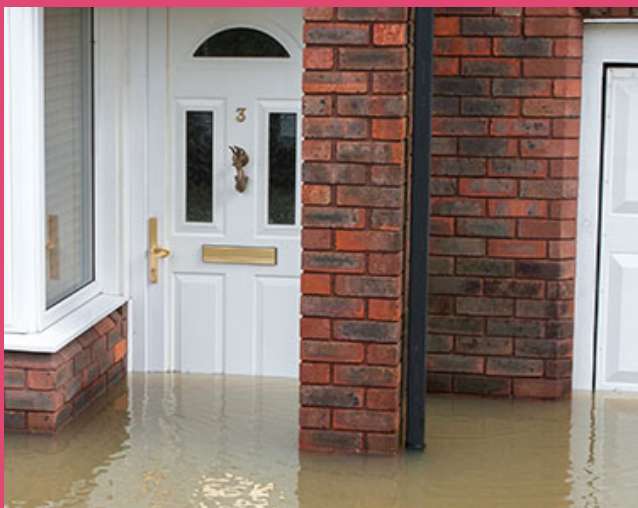
Source BRE Flood resilience. Masonry construction suffers less damage
